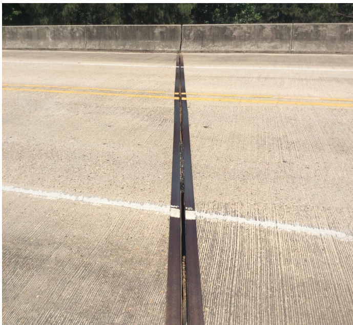
PHOTO 1 Description Bent 2, 8' of joint material missing.
